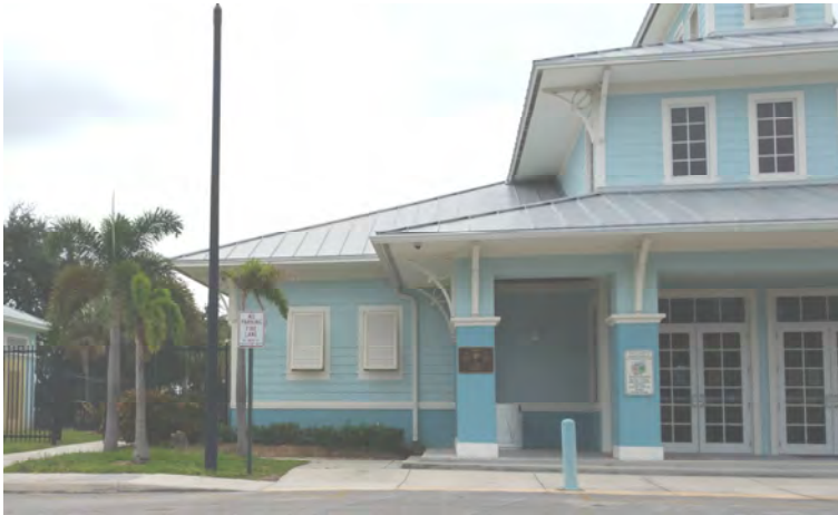
The existing building could be renovated to a Tropical design similar to other park buildings
