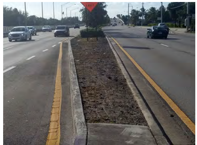
Median landscaping is difficult because space constraints limit variety and health of plantings
