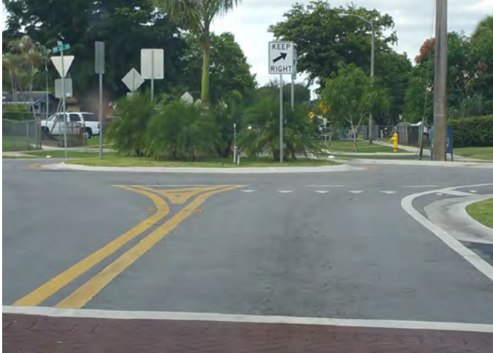
New roundabout installed on NW 34 Avenue
