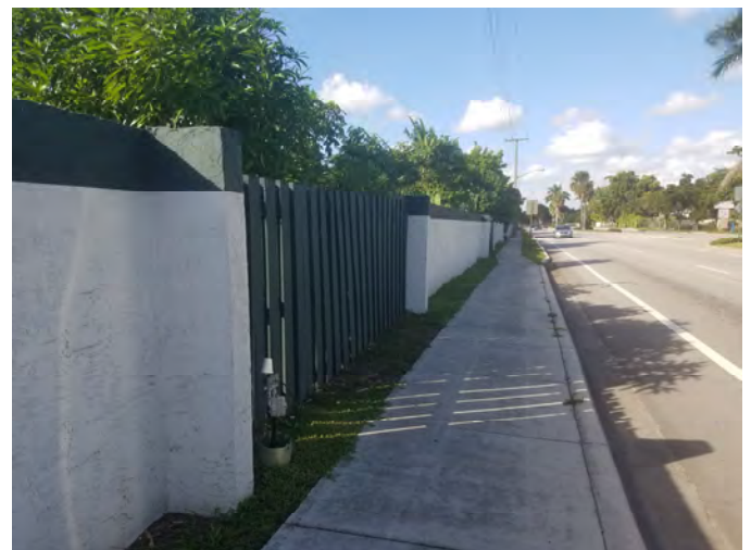
Existing walls/fences at Estates of Inverrary to be replaced
