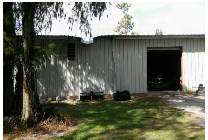
The existing maintenance shed will be demolished
