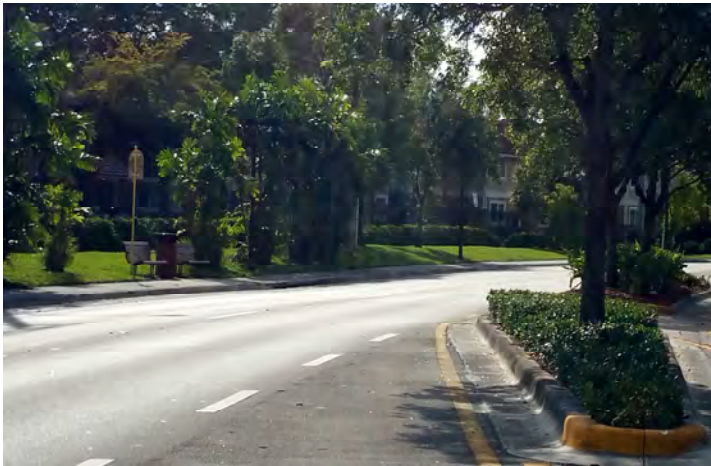
The NW 56 Avenue project from 2005 GO will be a model for the work planned for NW 47 Avenue
