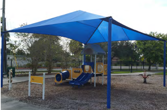
A new shade structure for playground will be installed
