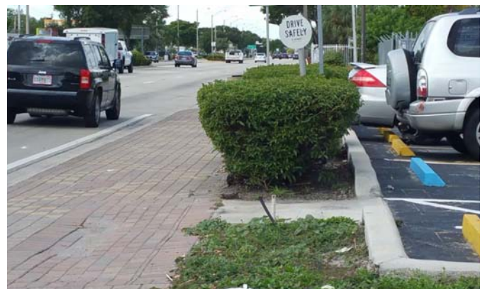
Space for landscaping and lighting improvements is constrained by existing development
