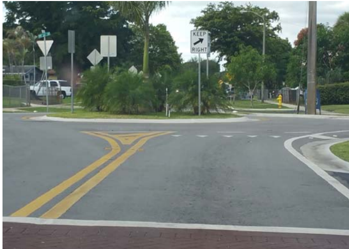
New roundabout installed on NW 34 Avenue
