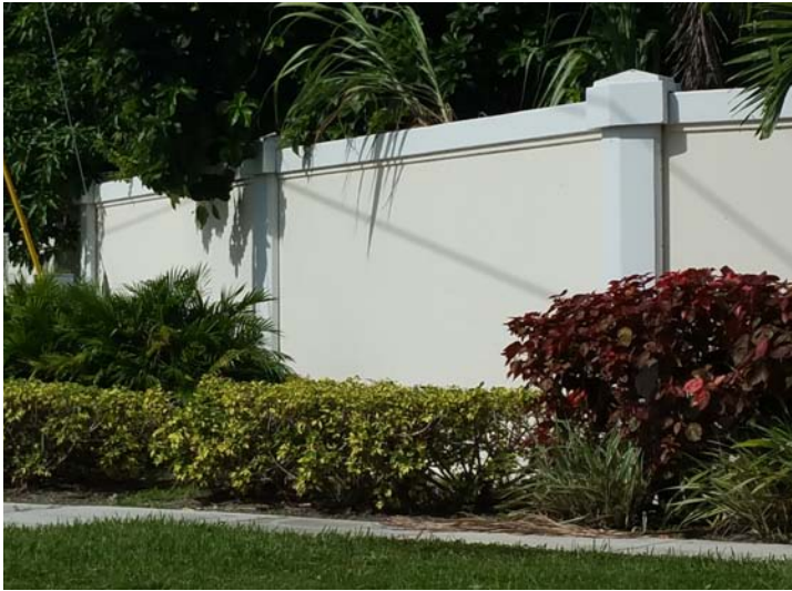
The new walls will follow the design used in 2005 GO project
