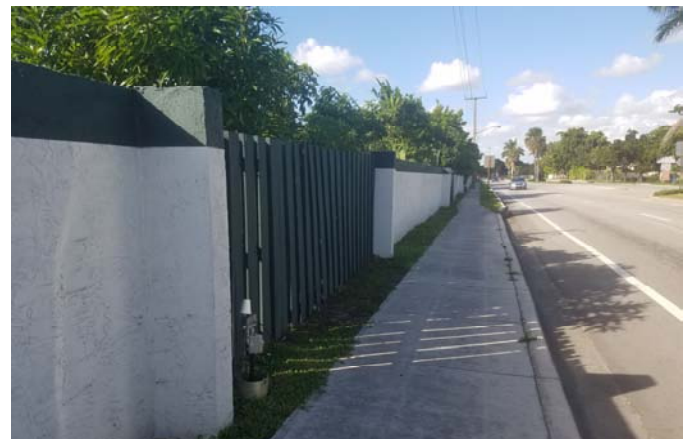
Existing walls/fences at Estates of Inverrary to be replaced
