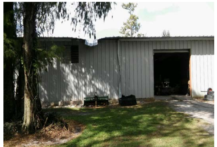
The existing maintenance shed will be demolished
