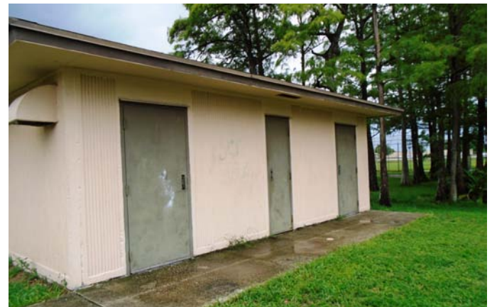
The restrooms at Mullin Park will be renovated
