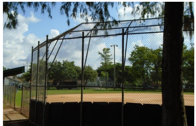
Renovation of baseball fencing and dugouts is planned for Veterans Park
