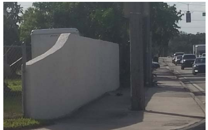
Existing wall at NW 19 St to be replaced
