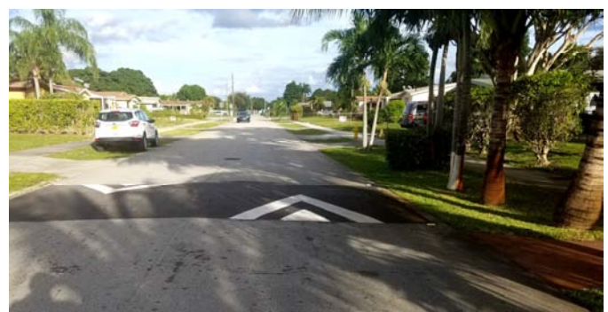
Speed humps are currently installed in many residential areas
