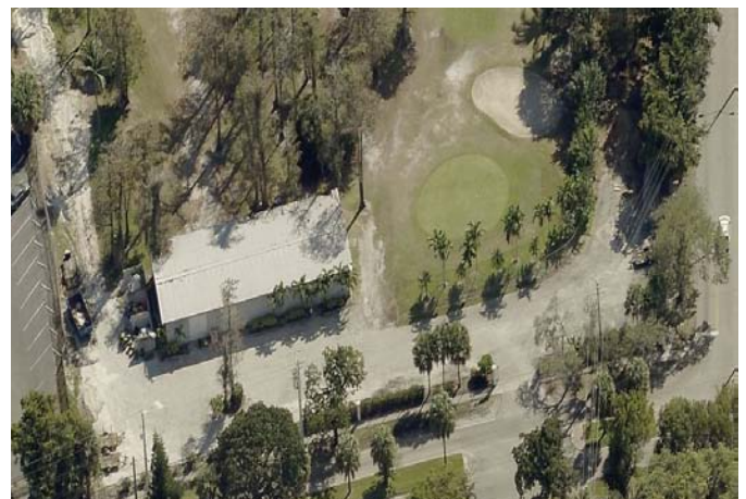
The existing maintenance shed will be demolished
