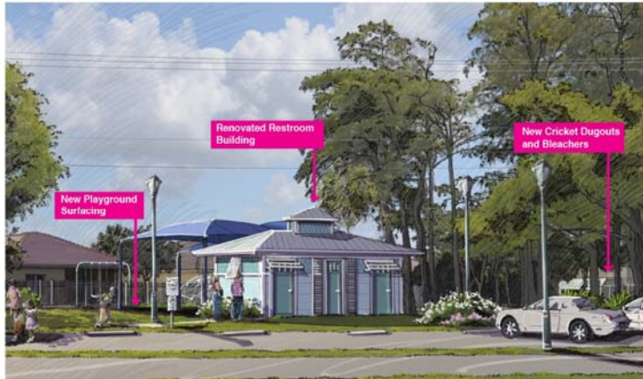
John Mullin Park Restroom Building - After Park, Recreational, Leisure and Cultural Projects
