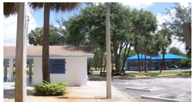
The Community Center will be renovated along with numerous improvements to the park amenities
