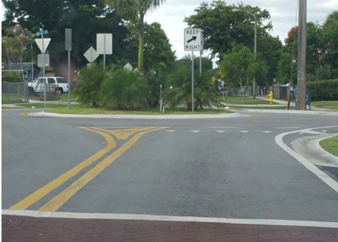
New roundabout installed on NW 34 Avenue
