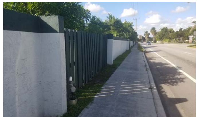
Existing walls/fences at Estates of Inverrary to be replaced
