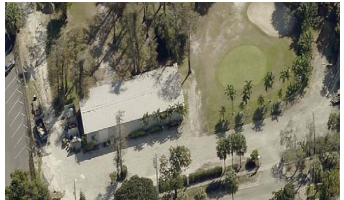
The existing maintenance shed will be renovated inside and out
