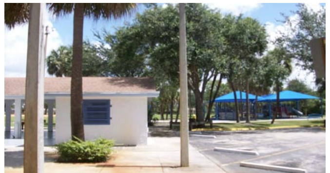
The Community Center will be renovated along with numerous improvements to the park amenities
