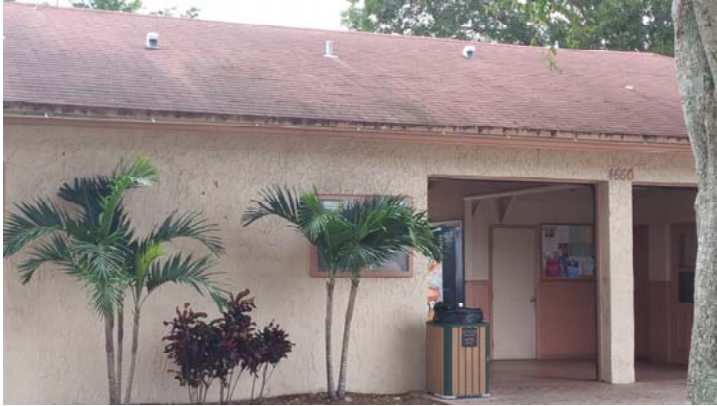
Staff is preparing cost estimates to renovate the existing restrooms or to add new restrooms to the building
