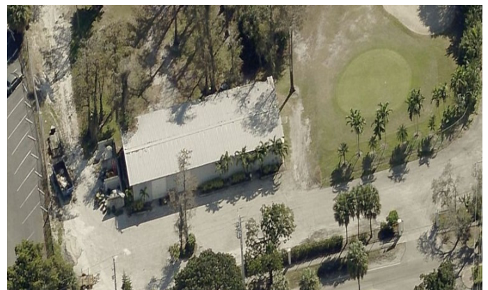
The existing maintenance shed will be totally renovated inside and out, making use of existing foundation and structural supports
