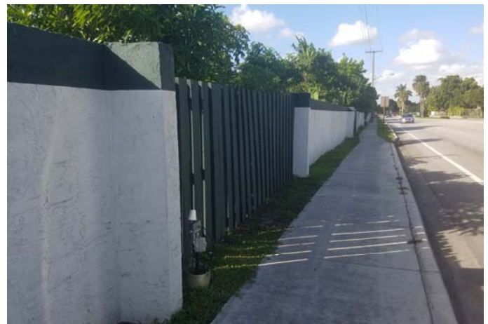
Existing walls/fences at Estates of Inverrary to be replaced
