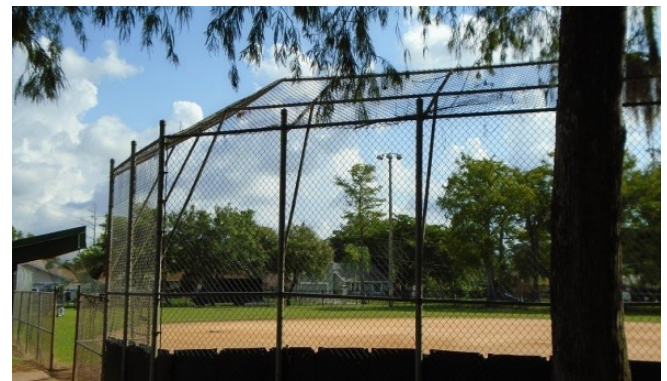
Renovation of baseball fencing and dugouts is planned for Veterans Park
