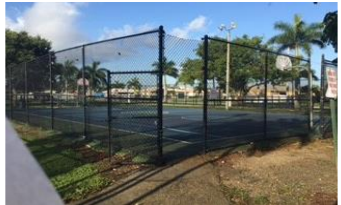
Westwind Park's basketball courts and fencing will be renovated
