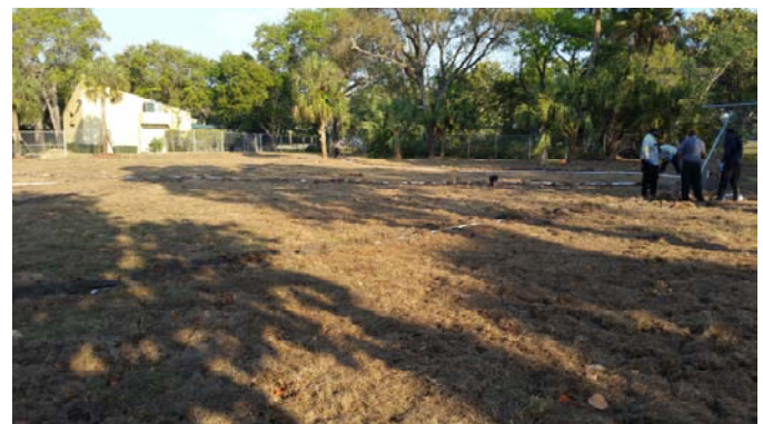
Demolition of the old Annex on NW corner of City Hall site was completed in February and the site has been restored with grass and irrigation
