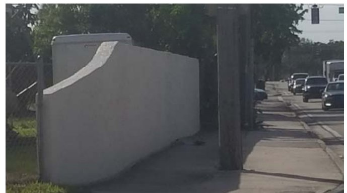
Existing wall at NW 19 St to be replaced at a future date
