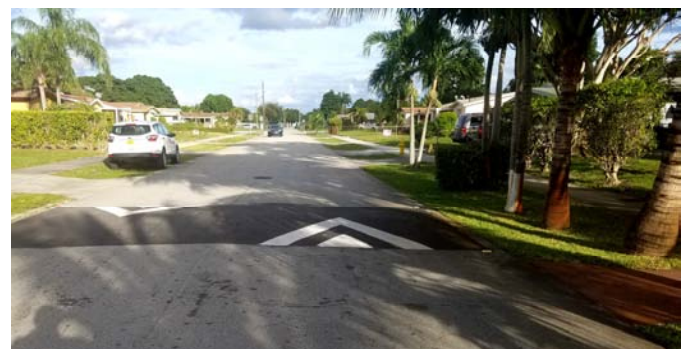
Speed humps are currently installed in many residential areas
