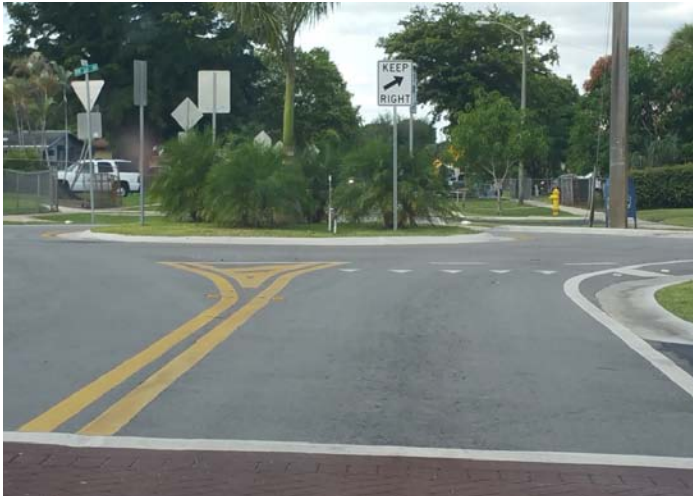
New roundabout installed on NW 34 Avenue
