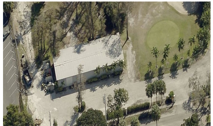
The existing maintenance shed will be totally renovated inside and out, making use of existing foundation and structural supports
