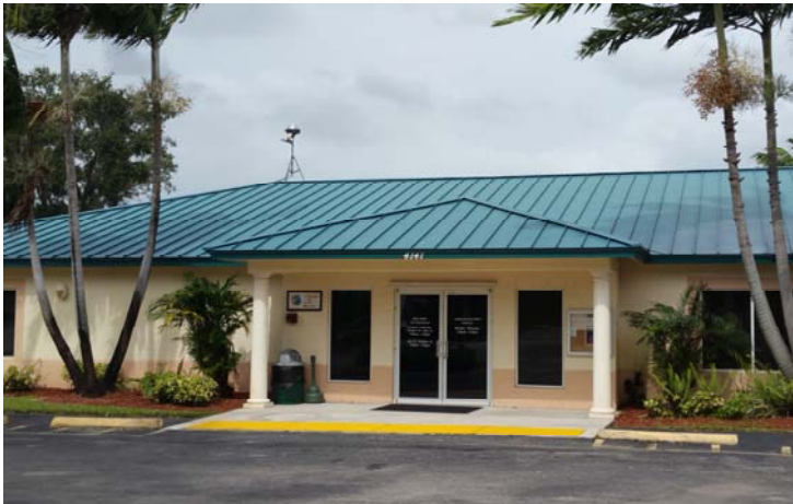
The renovated maintenance building will complement the existing clubhouse, which conforms to City design guidelines
