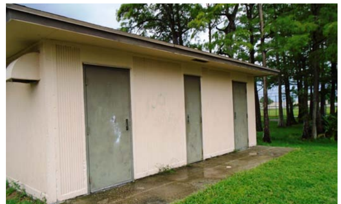
The restrooms at Mullin Park will be renovated
