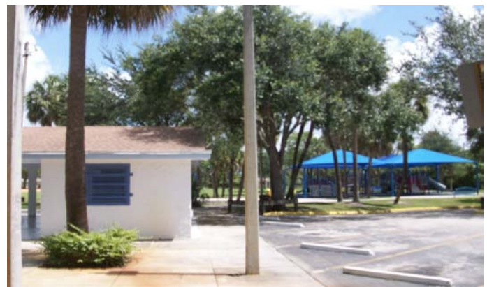
The Community Center will be renovated along with numerous improvements to the park amenities
