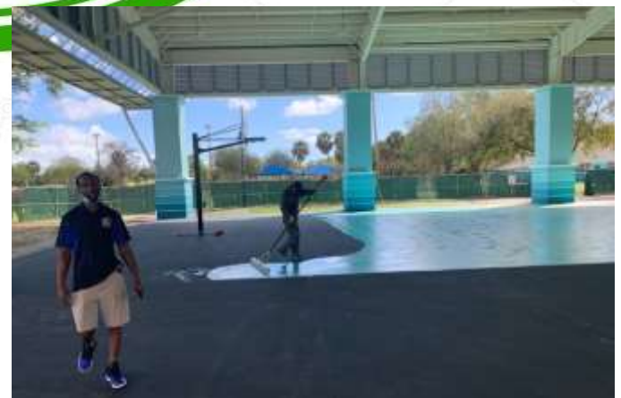
Basketball court floor will be completed early March, 2022
