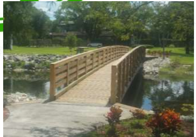
New bridge rails and decking have been installed
