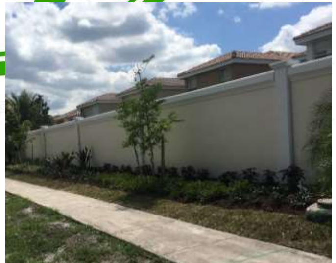
West Construction completed panel installation in 2019
