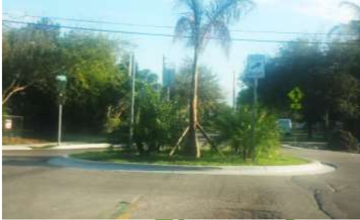
Completed Roundabout at NW 9 St & NW 34 Ave with new landscaping installed
