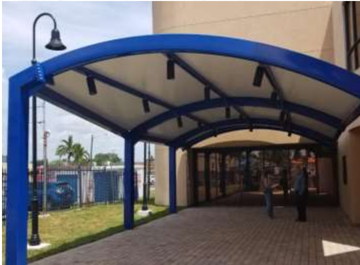
The new awning and paver patio has been completed on north side of building to provide space for outdoor activities
