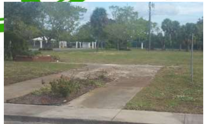
Saint George Church was demolished to clear the land for use in the redevelopment of the park
