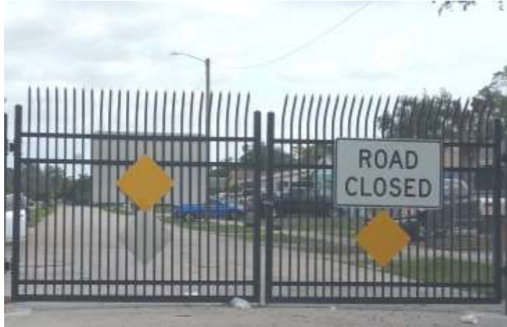
Fencing and gates installed at NW 33 Terrace to close road for vehicle and pedestrian access from Broward Blvd
