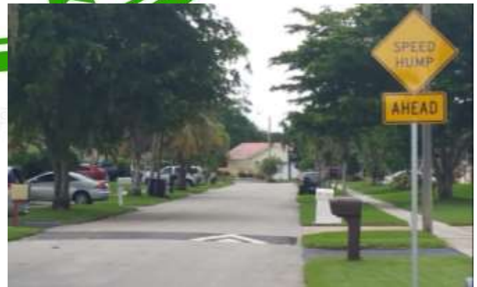
Speed hump installation has been completed at many new locations throughout Lauderhill
