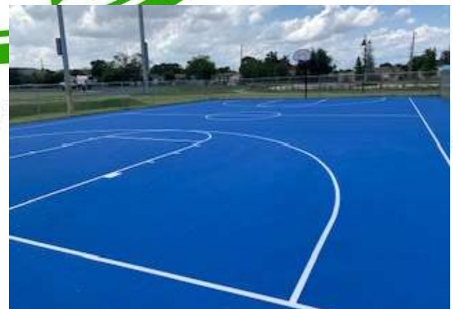
The new basketball court surface has been installed
