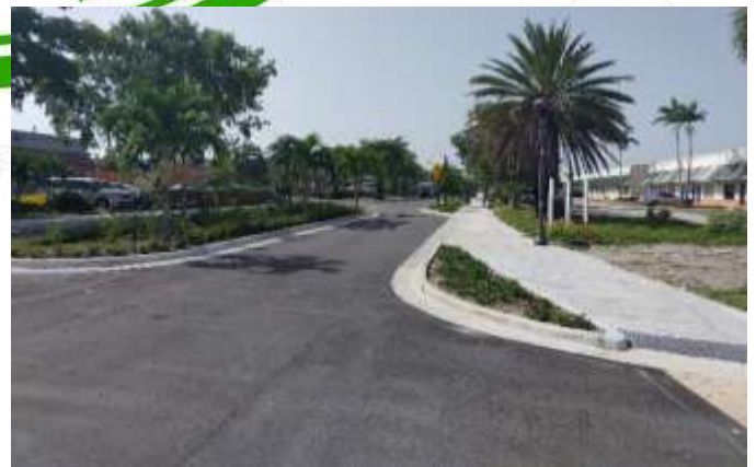
Final work is being completed on south end near NW 16 St
