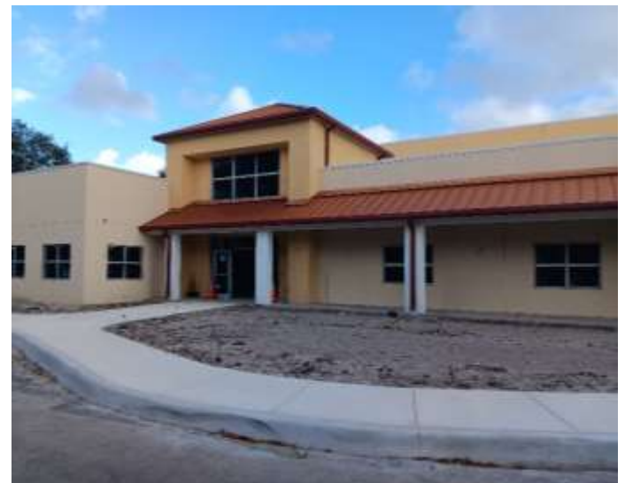
Ahrens Construction has completed the foundation and outside walls and begun interior buildout
