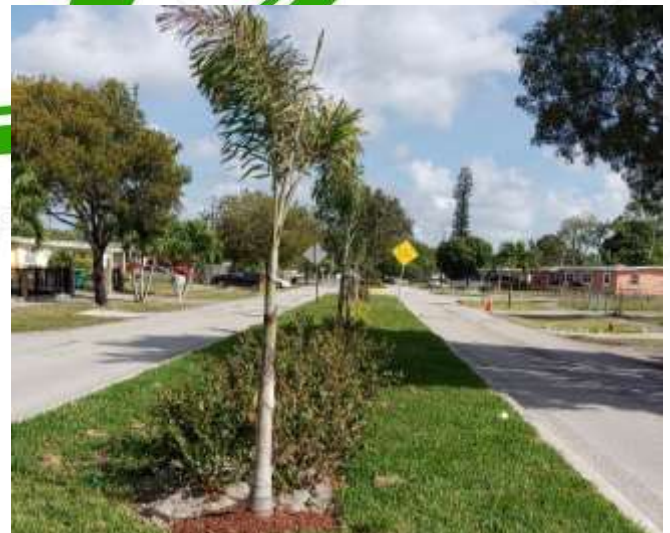
Improvements installed by City staff on NW 33 Avenue
