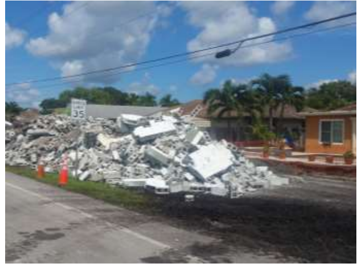
Rubble from the demolition of the old walls on NW 44 St
