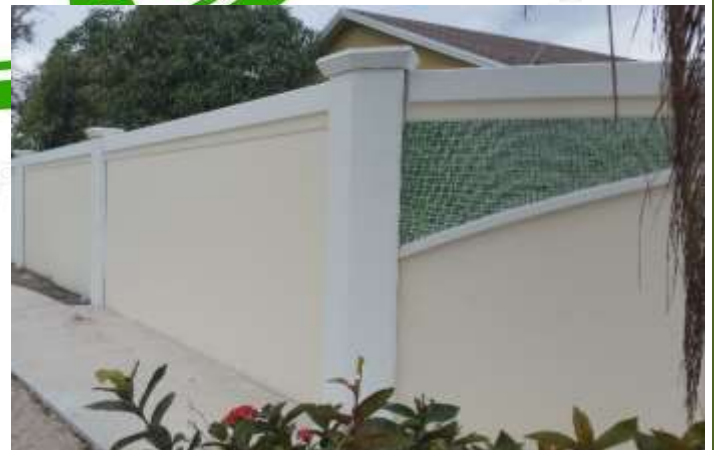
The wall panels, caps and decorative elements have all been completed
