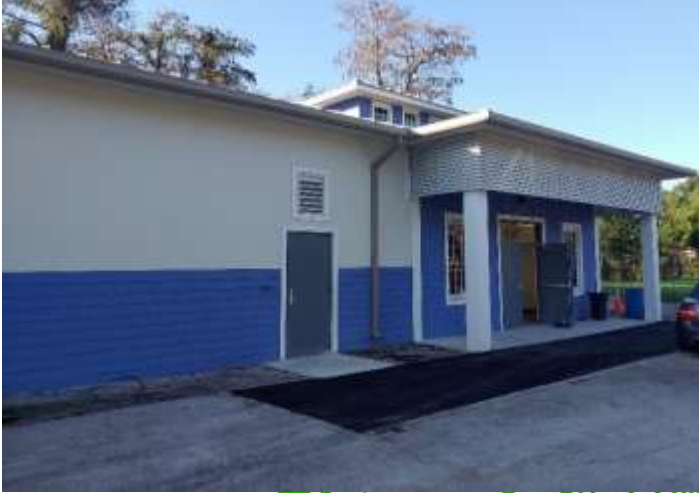
West Construction has completed exterior finishes and is completing interior buildout and painting.
