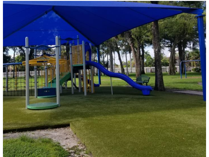
A new synthetic surface was installed beneath the playground that will reduce maintenance requirements and provide a safer play area
