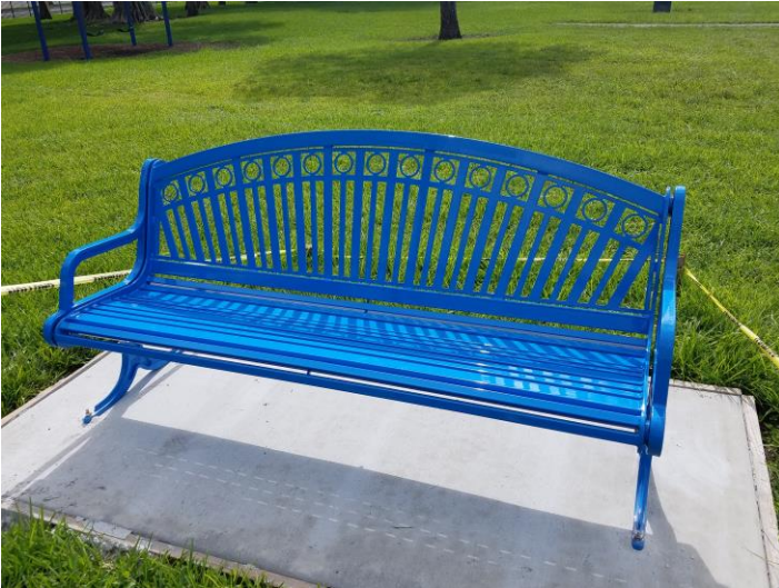
New high-quality steel benches and trash receptacles were installed on concrete pads
