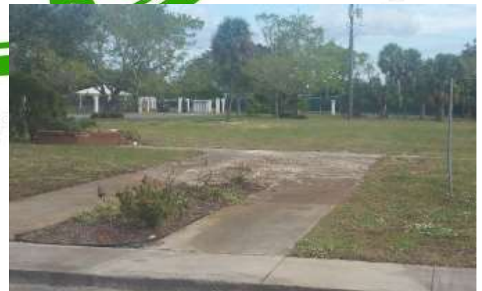
Saint George Church was demolished to clear the land for use in the redevelopment of the park
