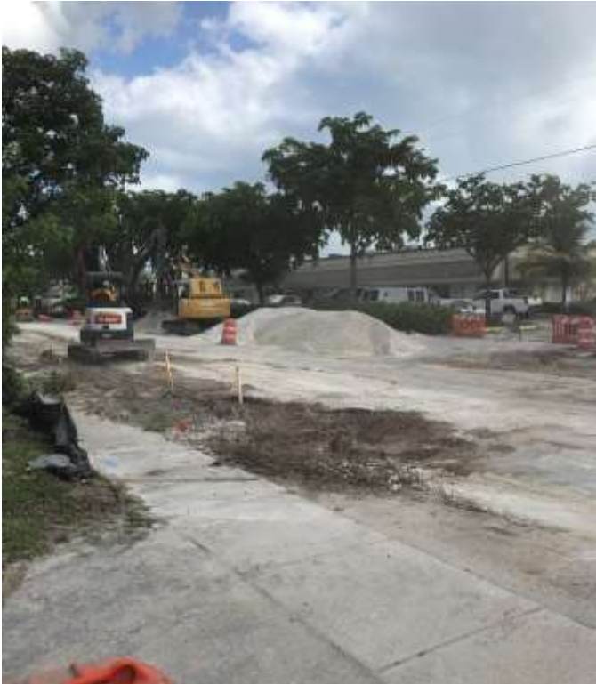
Installing new gravel base for roadway
