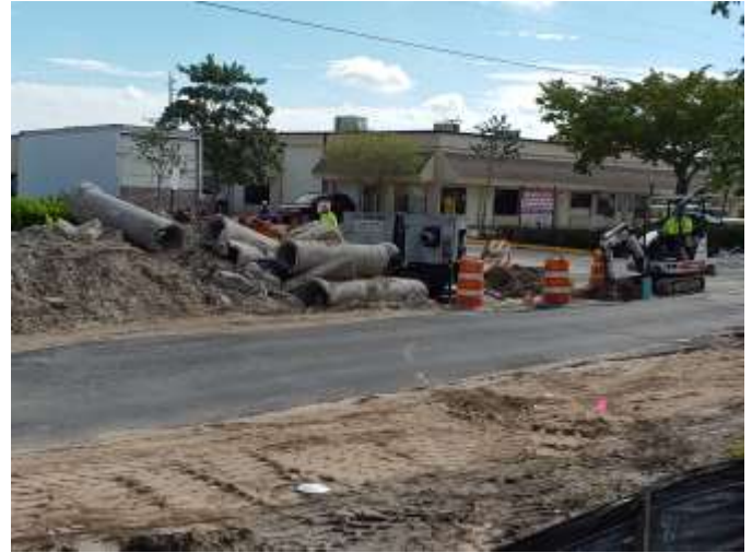
New water, sewer and storm drain lines
