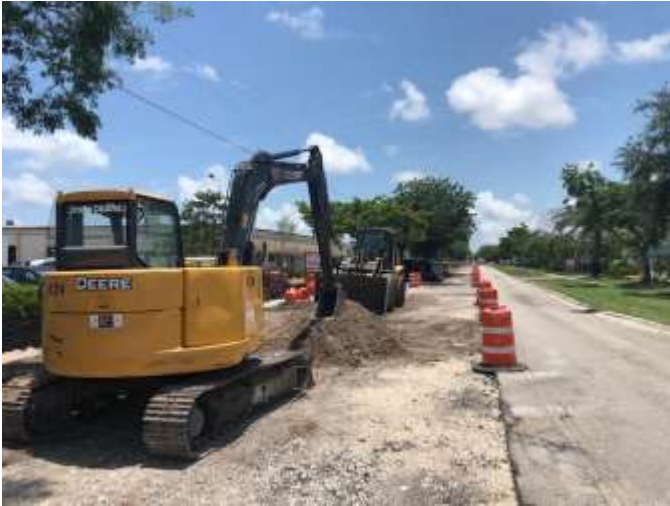
Removal of existing street and swales
