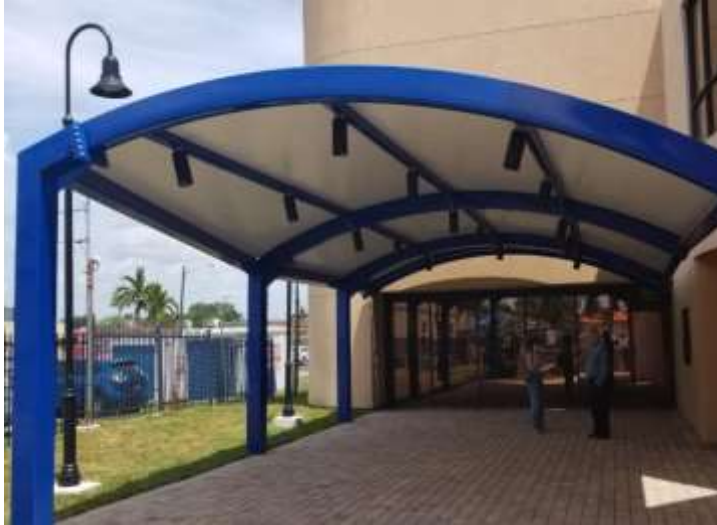
The new awning and paver patio has been completed on north side of building to provide space for outdoor activities
