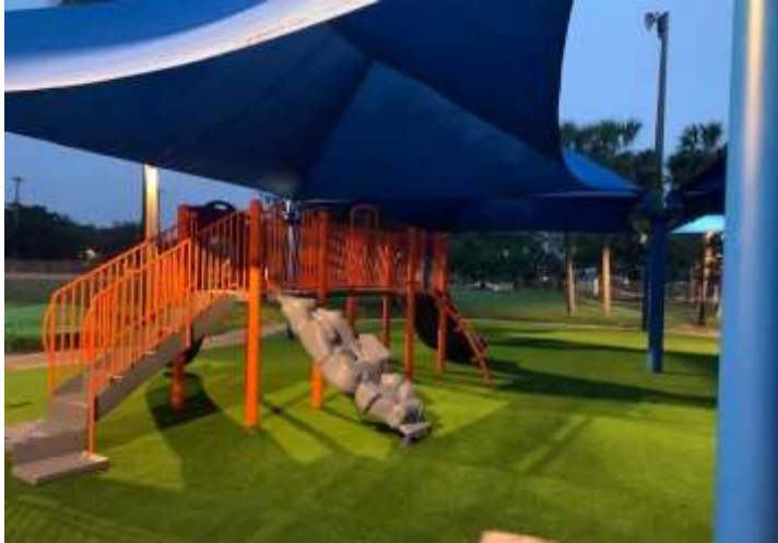
The new playground installation is complete
