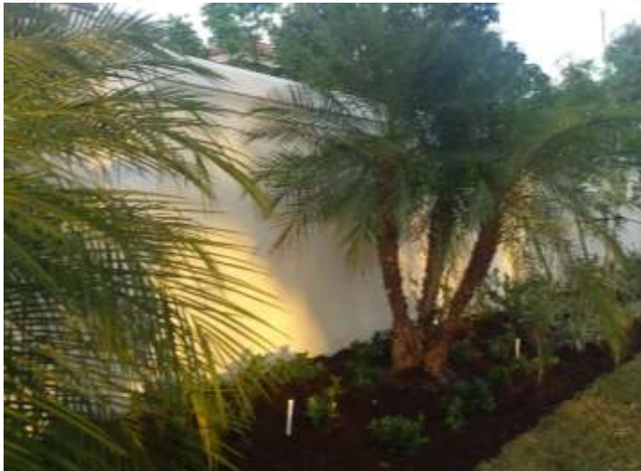
West Construction has completed the landscaping and irrigation installation along the new wall
