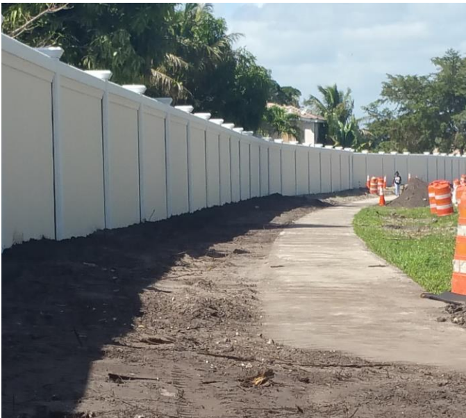
The wall panels and posts are topped with a decorative rail and caps
