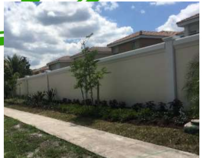
West Construction completed panel installation in 2019
