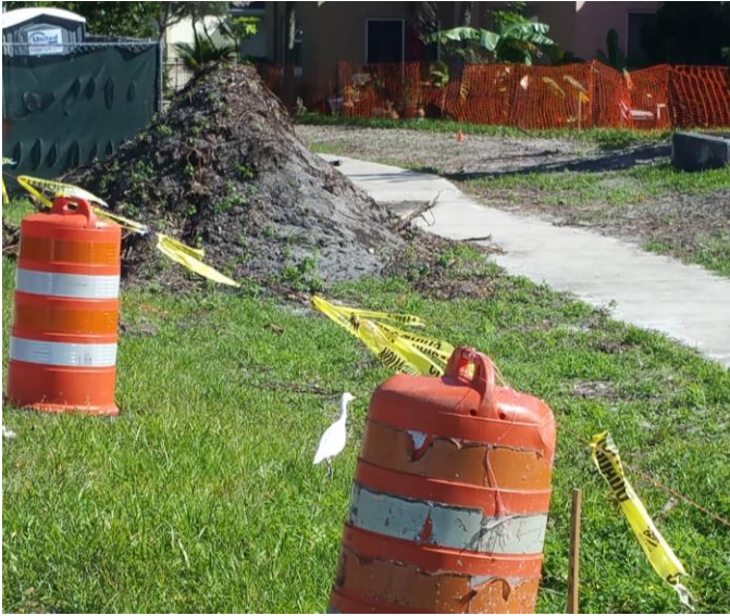
Construction began with the removal of the existing ficus hedges
