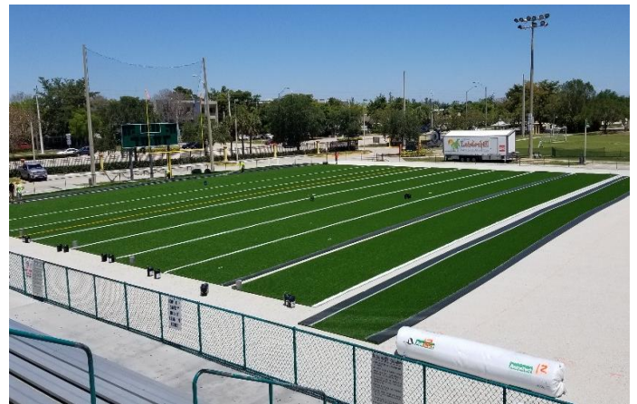
Field turf installation in progress over the prepared subsurface
