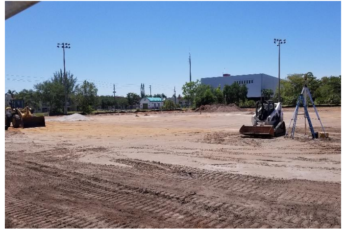
Grading the site to the proper depth and pitch is essential for playability and drainage
