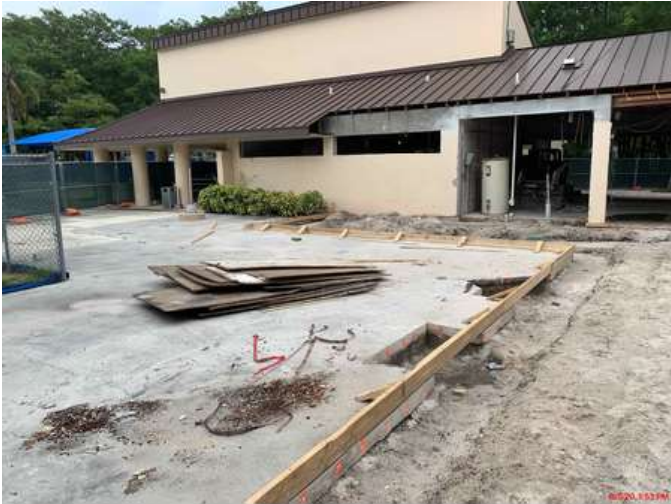
Photo of exterior renovations in progress
