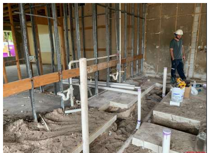
Restrooms and the kitchen are also being upgraded
