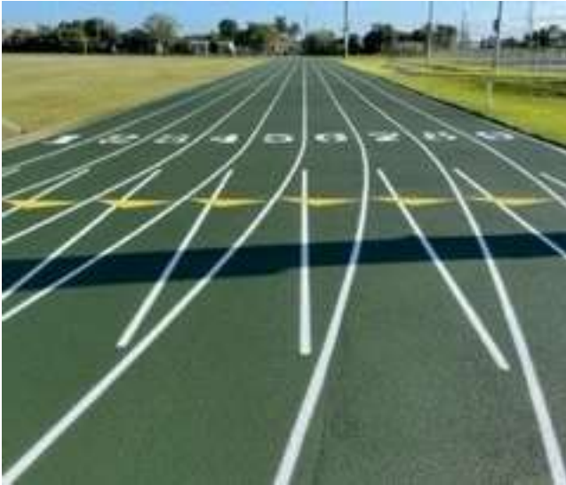
The running track installation and striping is complete
