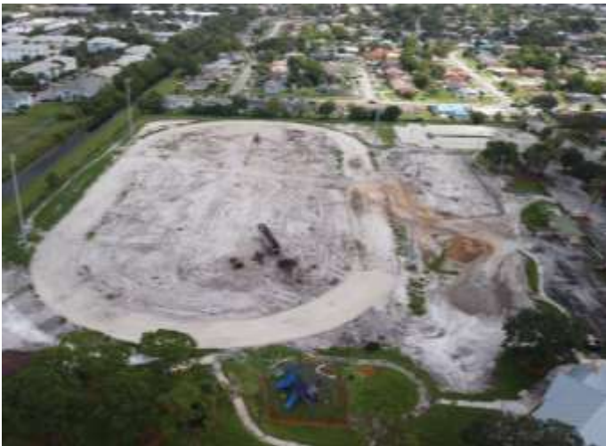
Aerial photo of West Ken Lark Park during construction
