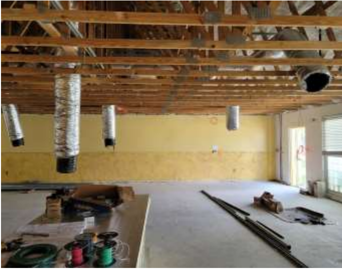
Interior renovations to building
