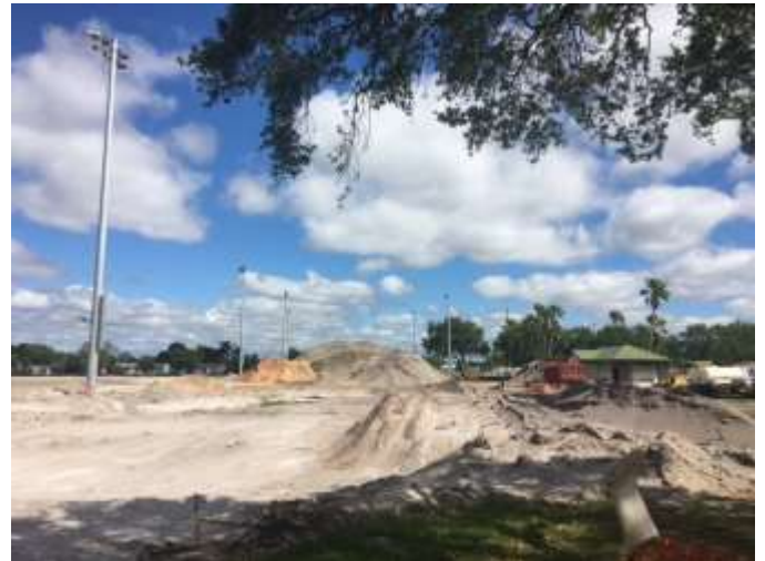
Earth moving prior to construction of improvements and running track
