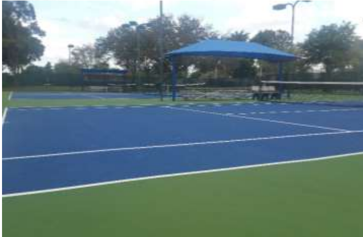
The tennis courts and basketball courts resurfacing have been completed
