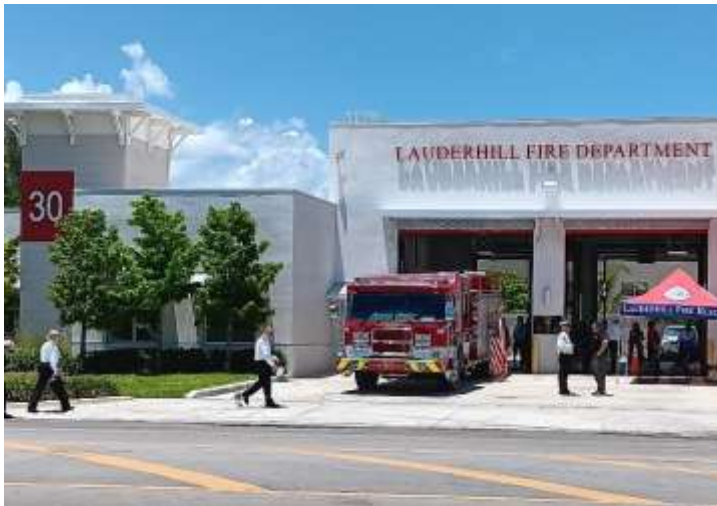
Newly-renovated Station 30 is located on 16 th St north of Lauderhill Mall and serves East Lauderhill
